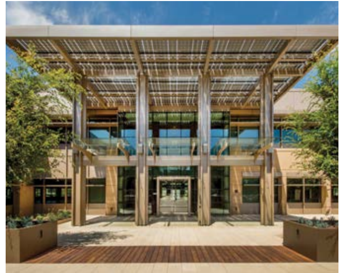
Entry way at Hanover Page Mill, Palo Alto, covered in solar panels. Credit: Devcon
