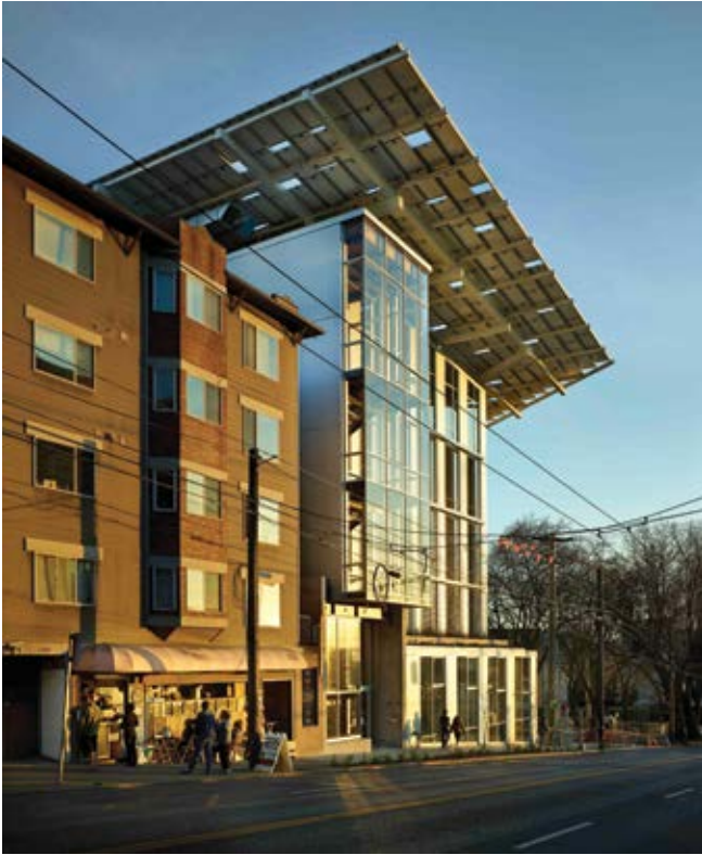
The six-story net zero energy Bullitt Foundation in Seattle. Credit: Benjamin Benschneider
