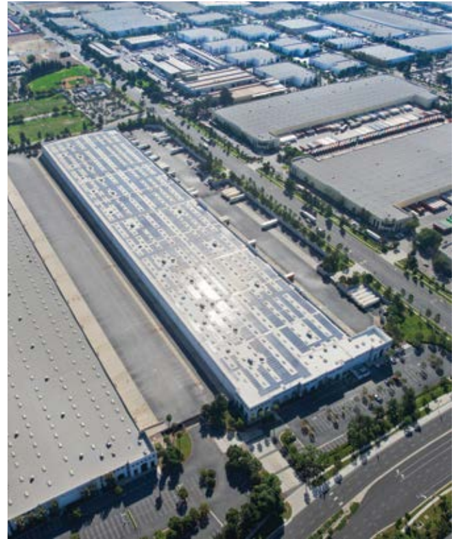
A 2.27 megawatt solar installation completed in 2015 at Prologis Rancho Cucamonga Distribution Center 1, Rancho Cucamonga, CA. © Woody E. Photography 2015.
