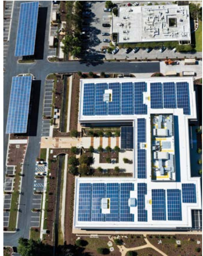
Credit: Steve Proehl Sun Light & Power
