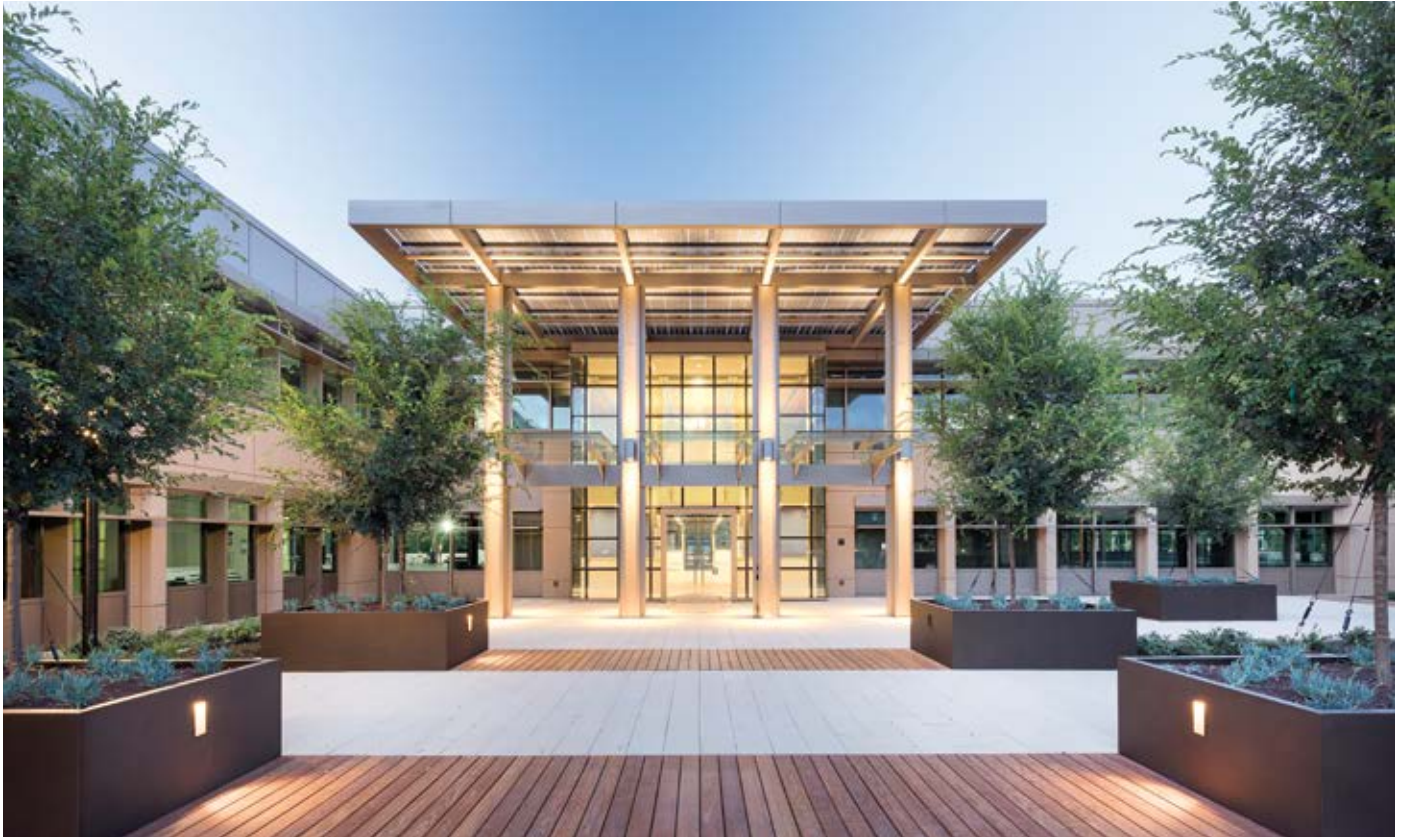
Entry way at Hanover Page Mill, Palo Alto, covered in solar panels. Credit: Eastdil
