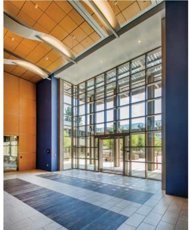
Lobby of the Net Zero Energy 1400 Hanover Page Mill office building. Credit: Devcon
